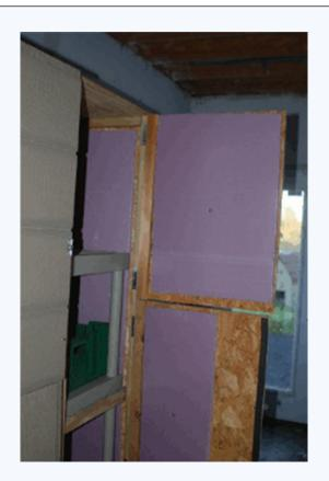
Note the insulation foam inside the cabinet, which keeps out both excess cold and heat. I cut a hole in the back to allow the dryer vent to exit. Behind the unit is a window. I closed it off with a piece of wood with a hole for the vent, then insulated it with spray foam.
